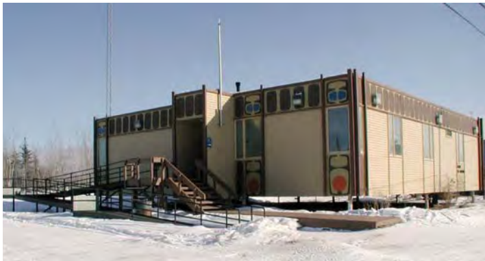
Fort Yukon Courthouse (Fourth Judicial District)
